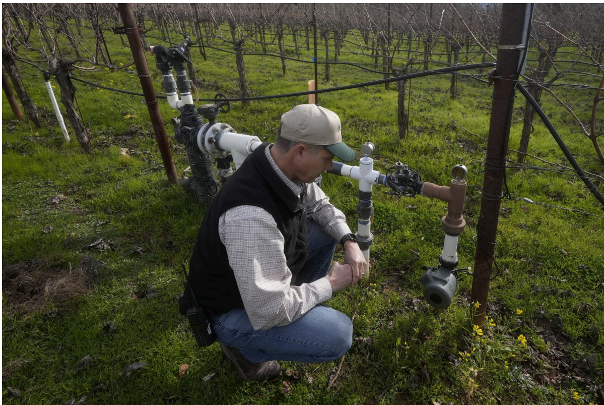
Fig. 6. Lumo smart irrigation valve in a Cabernet Sauvignon vineyard
